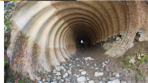
Failing Pipe
