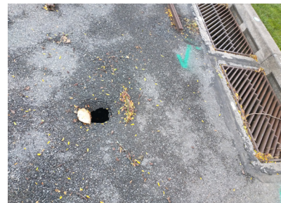
Failing Pipe
